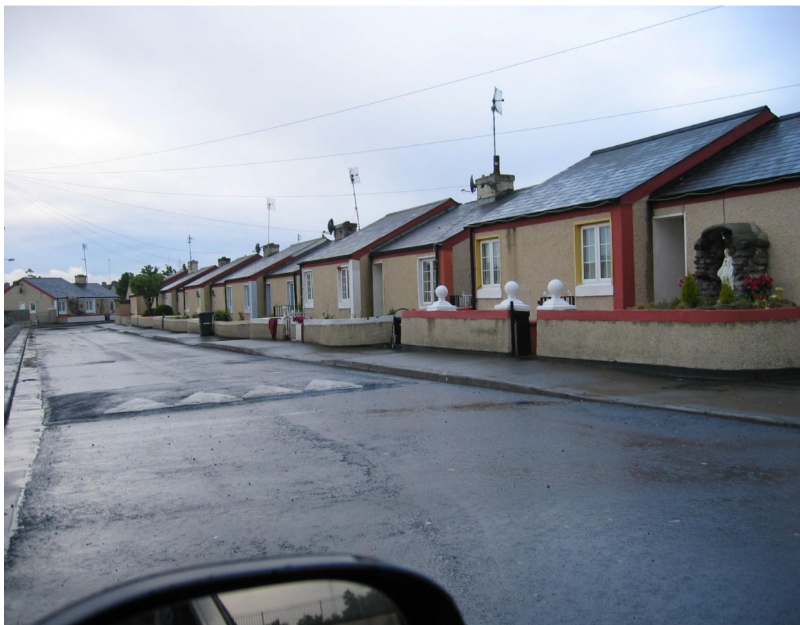
Cara Group Housing Scheme, Belcamp Lane, Coolock, Dublin 17
